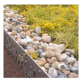
Washed Riverstone / Ballast is installed in conjunction with a loose laid protection fleece. A typical system application is a minimum 300mm wide and 85mm deep border, or according to system assembly. The border width should be
