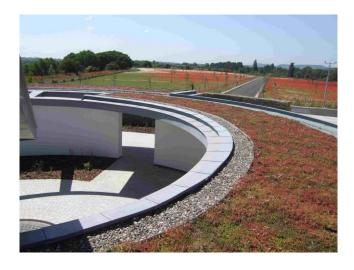
Extensive living roofs are not usually trafficked but are intended to be visual or ecological features. Typically, they have thin substrate layers to minimise depth and weight and are designed to be low maintenance with slow growing vegetation. They are often created to provide habitat for flora or fauna and to enhance building performance by reducing rainwater flow rates and increasing thermal efficiency.
