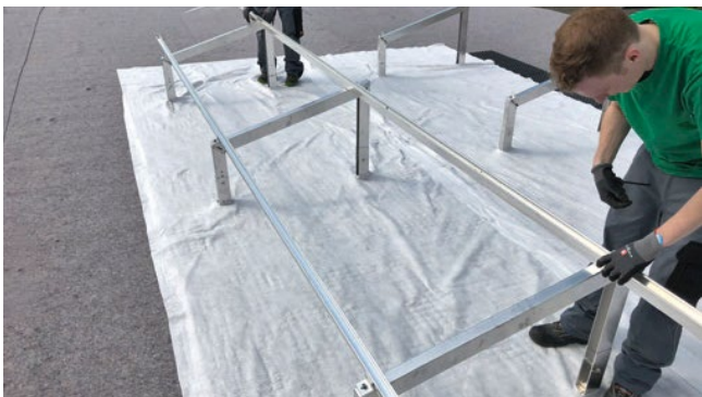
Figure 23: Mounting the second Easy Mounting Rail.
