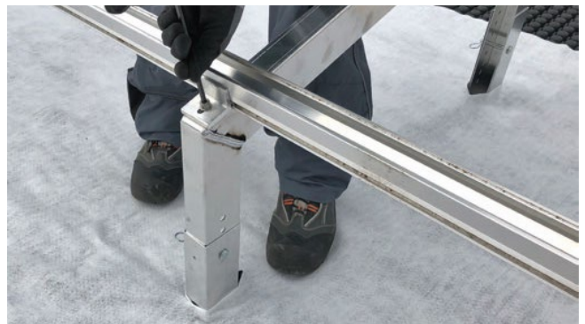
Figure 24: Tighten Rail Fixings.
