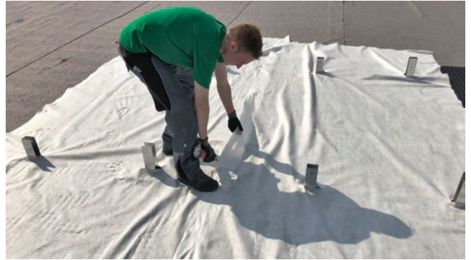
Figure 17 Bond rows of fleece with compatible adhesive.
