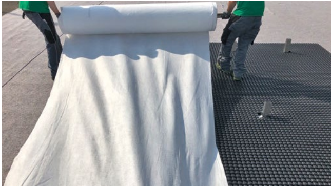
Figure 10: Rolling out the Filter Fleece.
