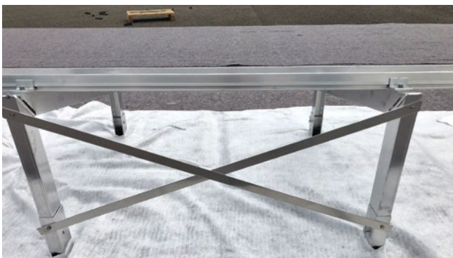
Figure 31: Wind bracing.
