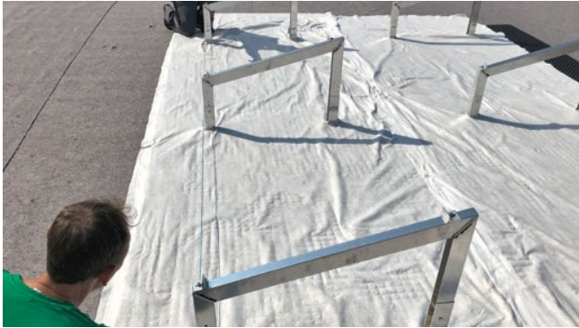
Figure 21: Alignment of the row using a string line.
