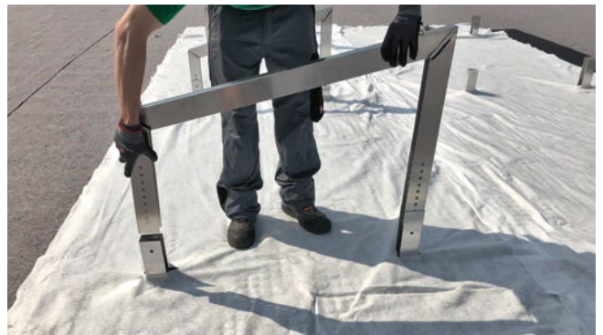
Figure 19: Installation of the Mounting Frame on the Base Plate.
