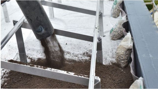
Figure 33: Blowing of the substrate.
