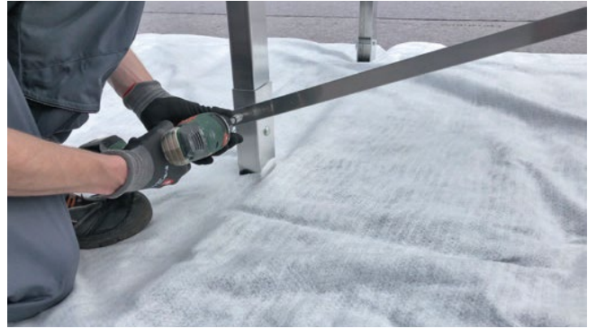
Figure 28: Fastening of the metal strip.
