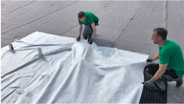
Figure 16: Lay second row of fleece.
