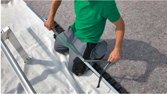
Figure 27: Removing the protective film from the wind bracing.
