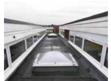
10 Rooflight Kerbs and Upstands
