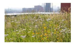
Extensive living roofs are not usually trafficked but are intended to be visual or ecological features. Typically, they have thin substrate layers to minimise depth and weight and are designed to be low maintenance with slow growing vegetation. They are often created to provide habitat for flora or fauna and to enhance building performance by reducing rainwater flow rates and increasing thermal efficiency.
