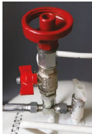
Image 9: Tighten the nut
